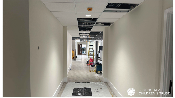
Progress at One Avenue Road
